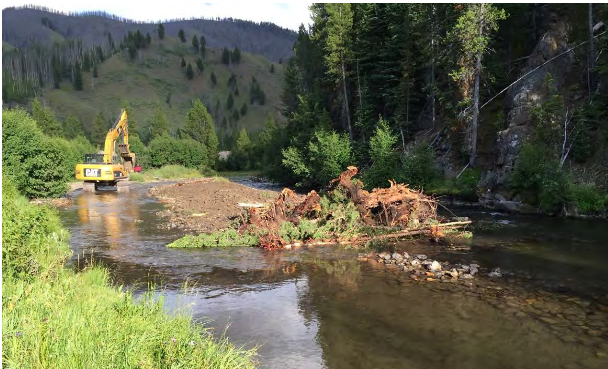
Figure B.17 Example photo of mid bar-forming ELJs.
