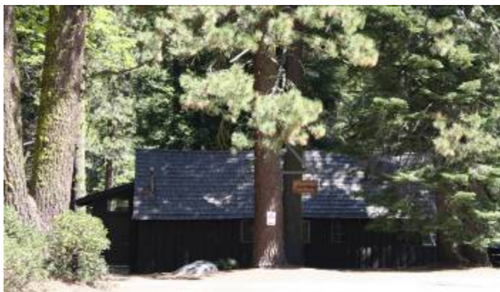
Figure 2-2. Building at Crane Flat Campus
