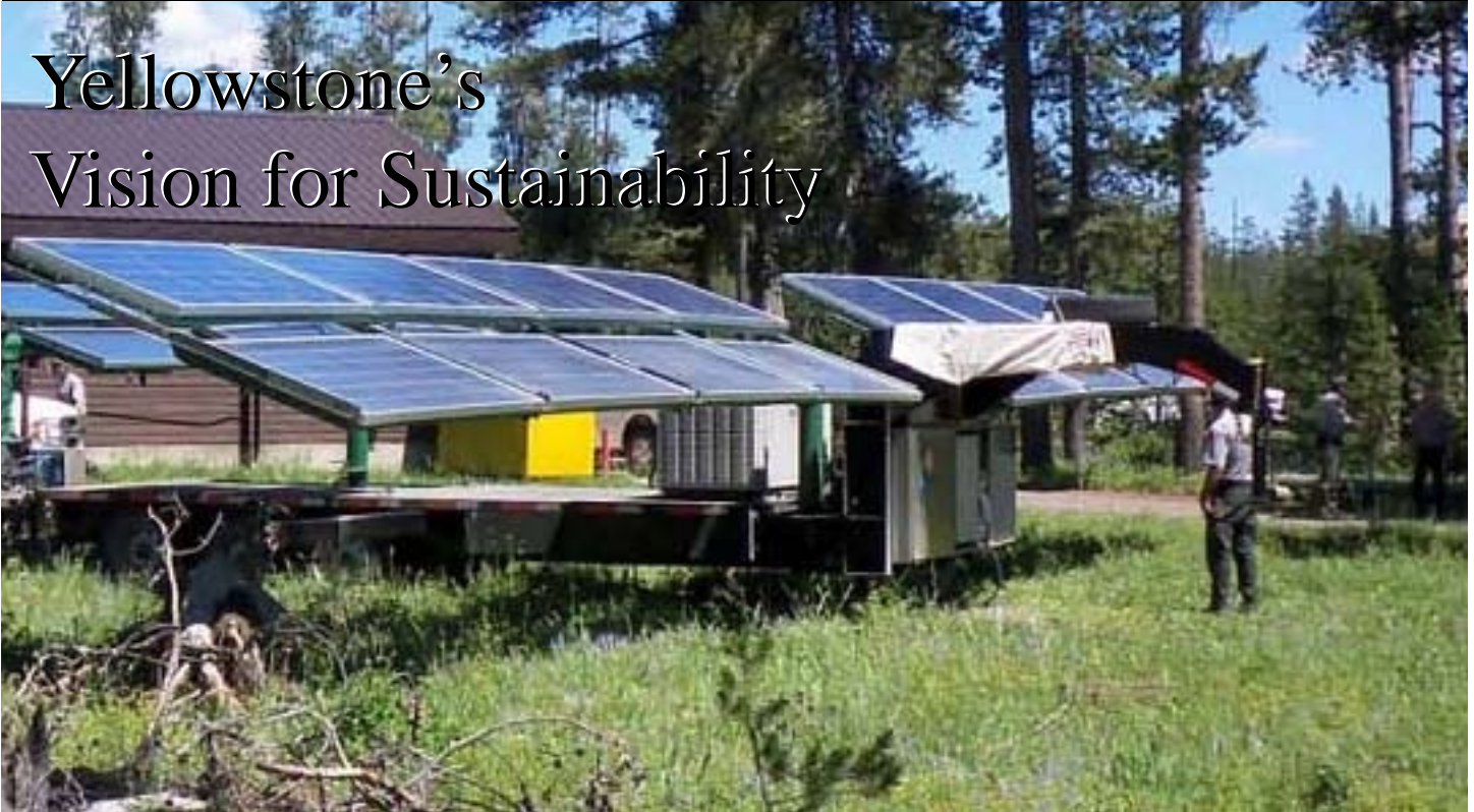
A portable solar array provides power at the Bechler Ranger Station in the summer season.
