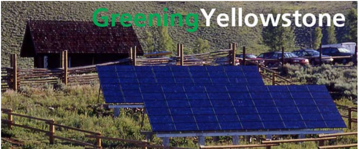
Lamar Buffalo Ranch's electricity comes from photovoltaic panels.
