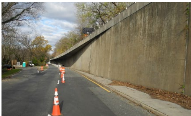
Figure 16. Cantilevered portion of the Clara Barton Parkway (Source: NPS)
