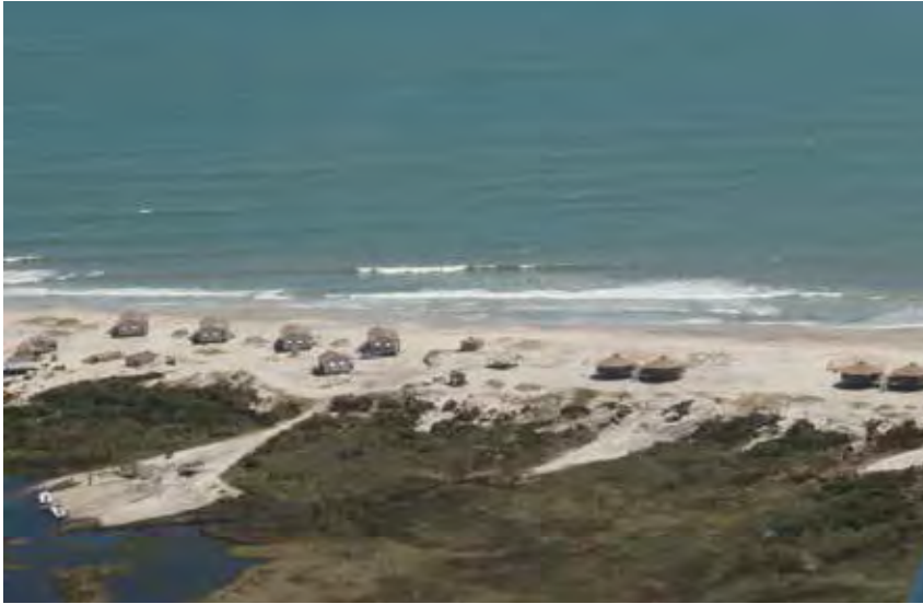
Overwash during Hurricane Irene impacted infrastructure on Long Point. Image credit: Rebecca Beavers, NPS.
