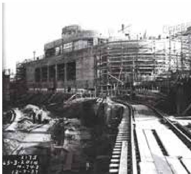
**Figure 19.** WPA photograph showing the relocated State Belt Railroad tracks, extent of excavations, and by the end of 1937, progress on construction of the Bathhouse. View looking southeast. (*San Francisco Maritime NHP, Historic Documents, Photograph Collection, P88-035.00106*)
