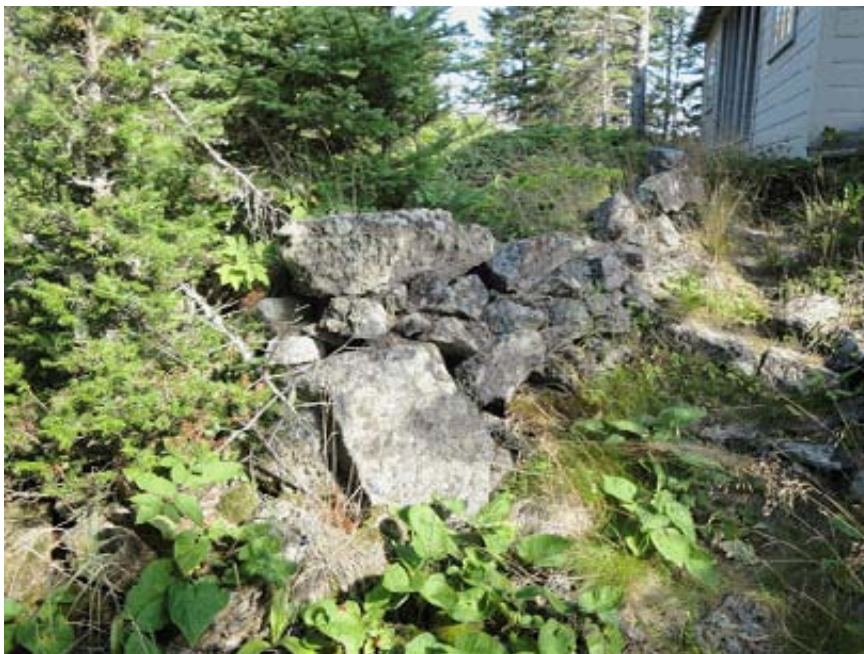
Stack Retaining Wall (Jackson 2010)
