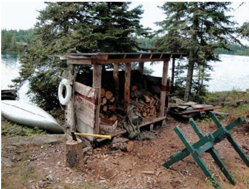
Gale Firewood Storage Shelter (Jackson 2010)
