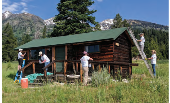
Volunteers preserve the wood by applying linseed oil at the historic White Grass Dude Ranch.
