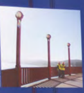
As the Bridge design evolved, consulting architect Morrow's touches included details in the popular Art Deco style, a thoroughly 20th-century style based on geometrical shapes. Morrow's touches included chevron-shaped fluting and sleek, angled light stands and curved I-beams. He also proposed dramatic decorative details that were eliminated during construction but added in 1988 for the 50th anniversary celebration.
