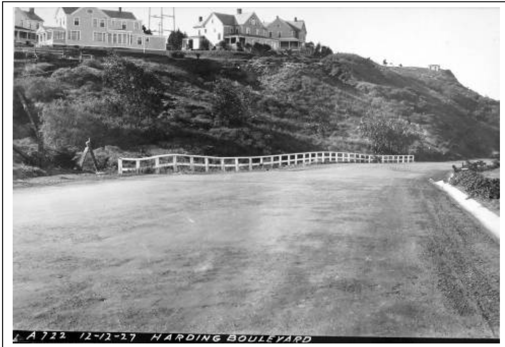
Figure 72. Roadway settling occurring below Fort Miley, December 12, 1927. (SFPL, DPW Coll.)
