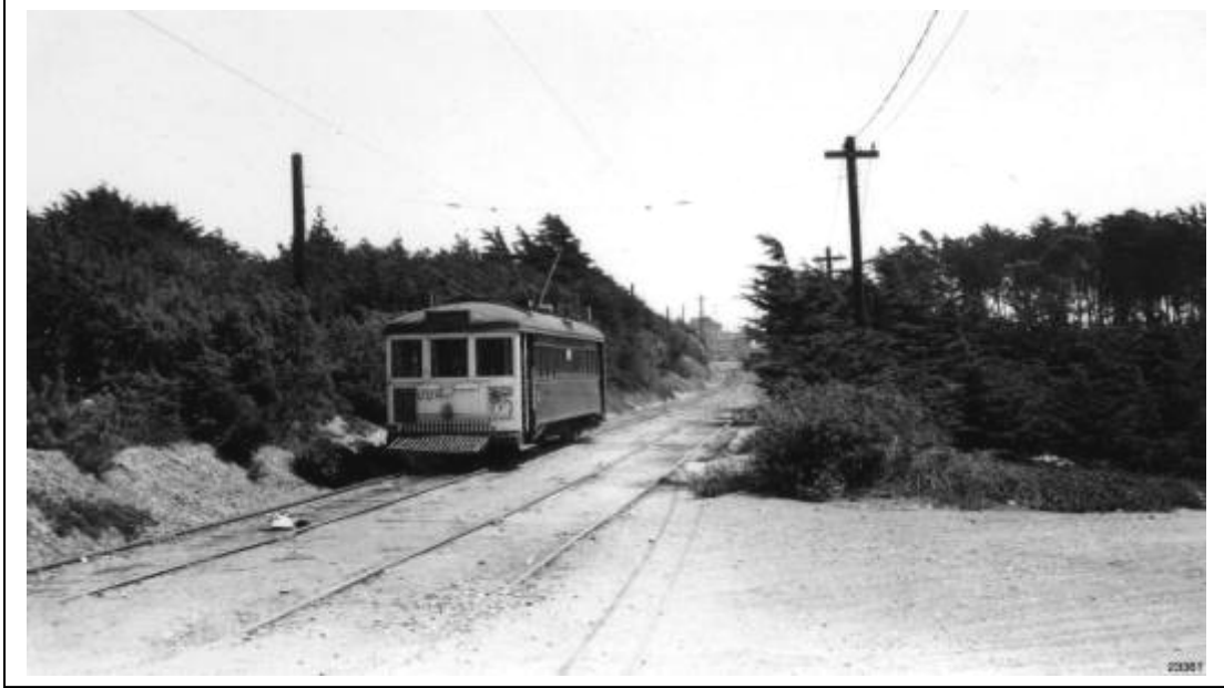
Figure 57. MUNI #1 car on private right-of-way at intersection with Merrie Way, August 1948. View southeast. The still-forested Triangle is at the right. (Bay Area Electric Railway Association)
