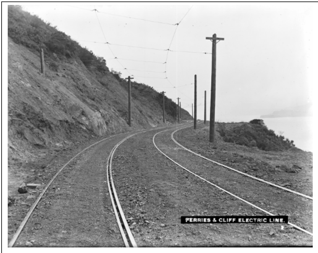
Figure 19. A section of newly-built streetcar track and overhead lines, May 1905. This stretch of line was located west of today’s Eagles Point. View looking west. (Municipal Railway, URR Ferries & Cliff Line series)
