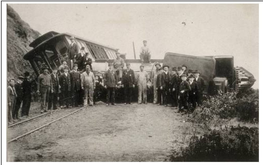
Figure 18. A bad day on the Cliff Line, February 2, 1901. (Bancroft Library)
