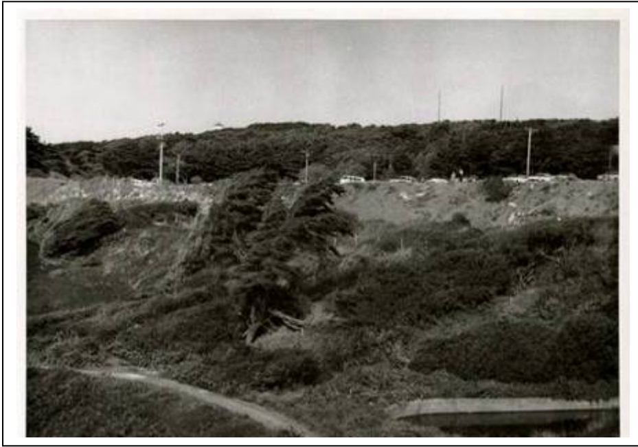
Figure 54. Fill dumped along the west side of Merrie Way, circa 1960. (SF Public Library AAC-0346)
