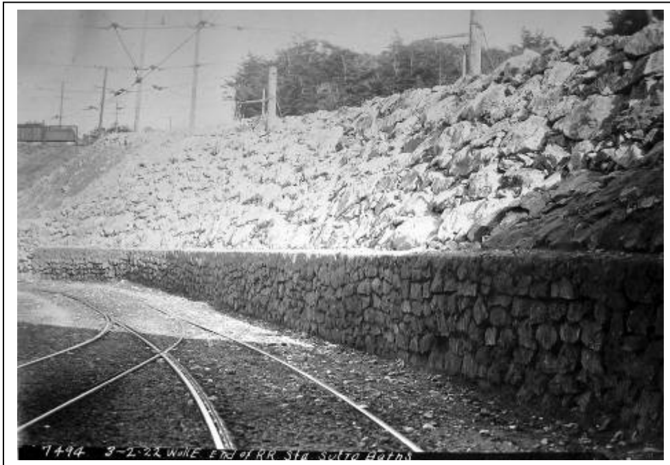
Figure 40. The rockwork wall constructed by the Department of Public Works to protect the streetcar tracks after Point Lobos Blvd was widened. (SF Public Library, DPW Collection)
