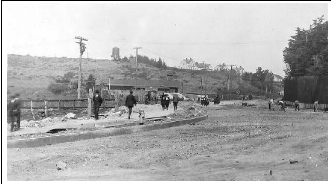
Figure 58. Repaving Point Lobos Avenue near Merrie Way on April 6, 1922. View north. The 48 th Ave. streetcar depot is visible at center. (SF Public Library, DPW Collection)
