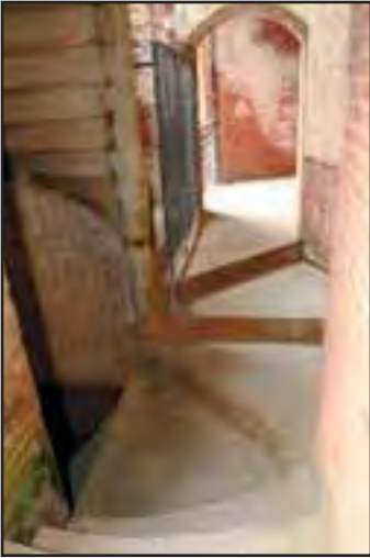
Each landing in the circular staircase is composed of slightly different shaped pieces of granite depending on the floor to floor heights. (John Martini, 2005)
