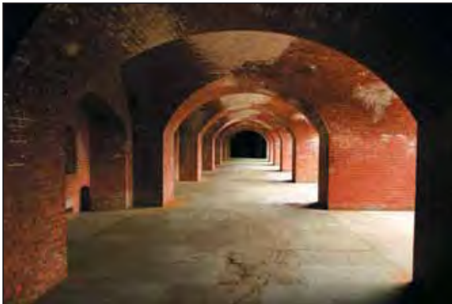
Typical brick casemates with arched ceilings and granite floors. (John Martini, 2005)
