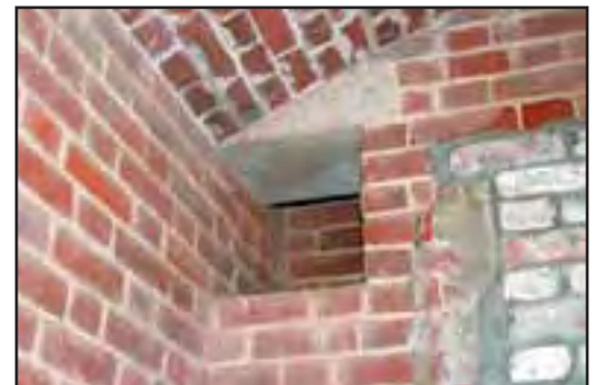
One of the square vents in the corner of each magazine with a small granite header. (John Martini, 2005)
