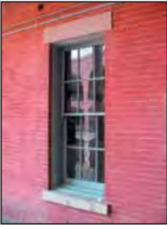
Typical wood frame window in gorge. (John Martini, 2005)
