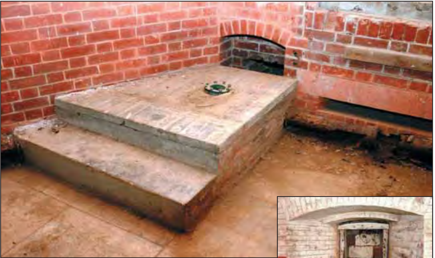
These concrete platforms for plumbing fixtures remain from the 1914 attempted remodel of the fort into a disciplinary barracks. (John Martini, 2005)
