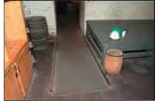
The reconstructed banquette on the right would have doubled as a platform to fire into the sallyport and a sleeping area for the guards. (John Martini, 2005)
