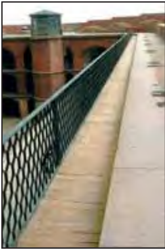
This 3-foot wide walkway and railing above the gallery on the southwest gorge elevation was replaced in a 1973 project. Beyond is the penthouse over stair #3. (John Martini, 2005)
