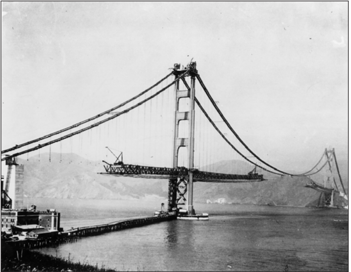
Figure 17. Photograph: Golden Gate Bridge construction, viewed from East, circa 1936. Credit: Fort Point NHS Collection, Golden Gate National Recreation Area.
