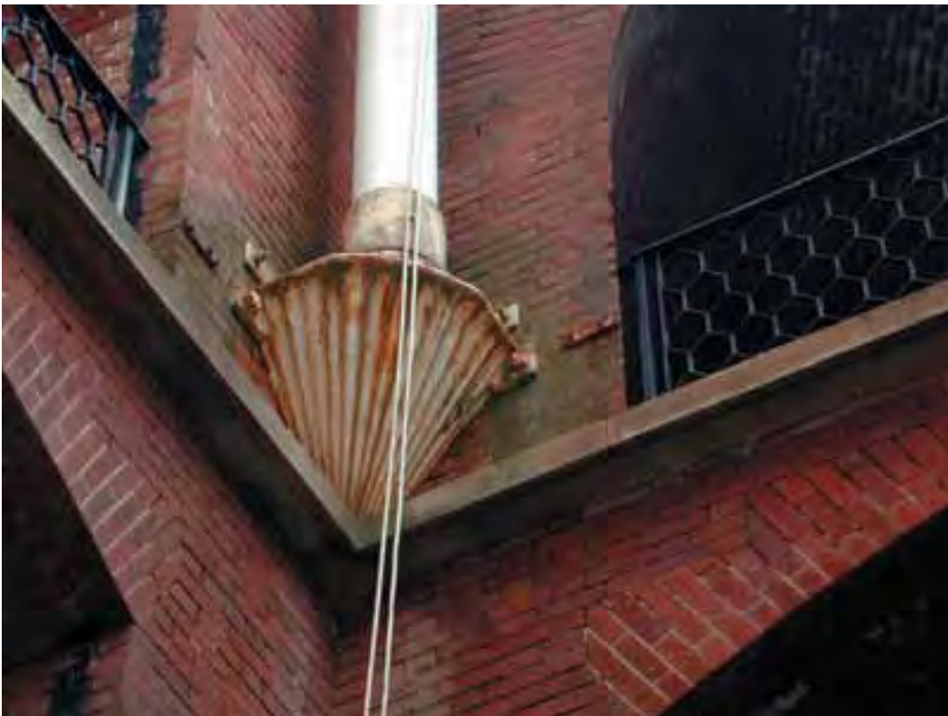
Condition Photo 11: Biological growth on flagpole. (Courtesy of ARG, 2003)
