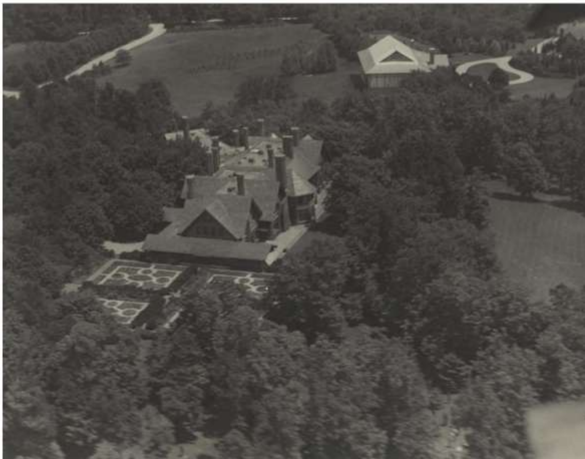
20. 10-5 D. DOWS, Muttontown / Brookville, Long Island, NY ("Charlton Hall")
