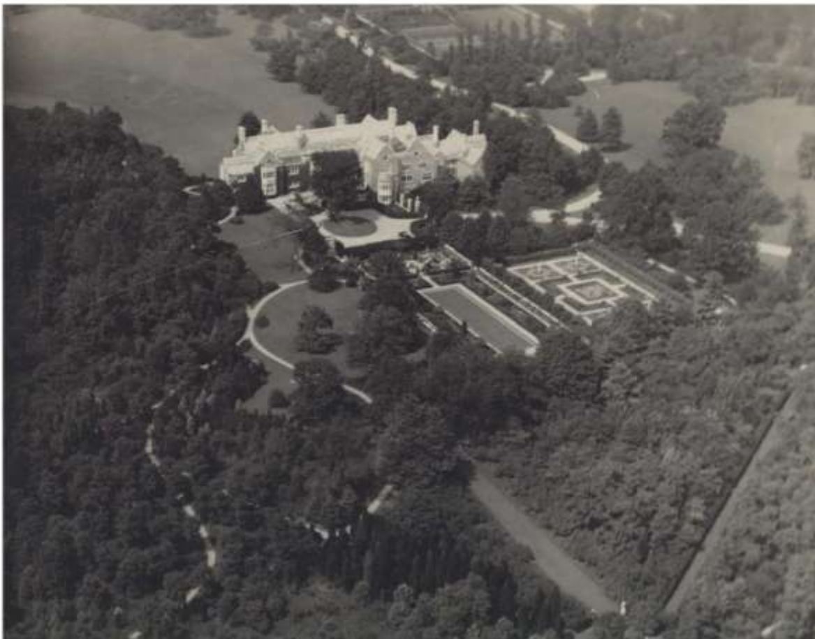
32. 13-3-5 ALDRED, Lattingtown / Glen Cove, Long Island, NY ("Ormston")
