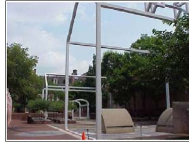
Example of ghost structure at Franklin Square, Philadelphia, PA.
