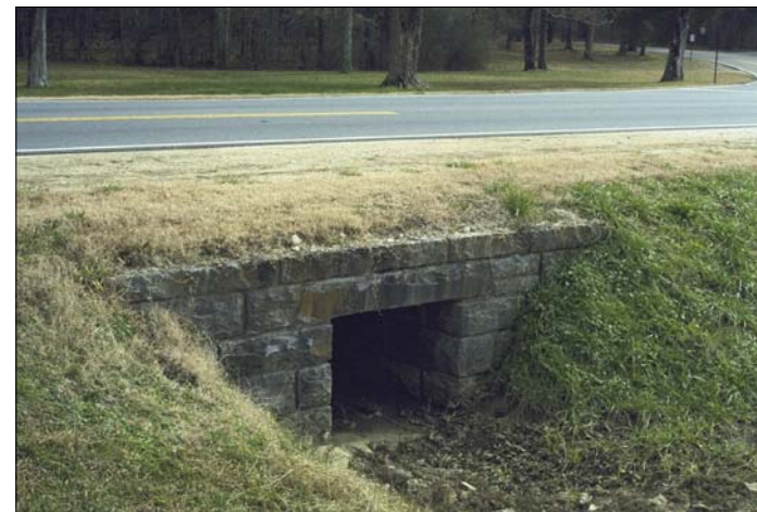
Example box culvert.
