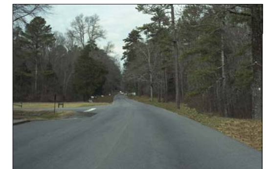
Same image edited to reflect the character of LaFayette road with reduced cross-section, less fill, and no striping.
