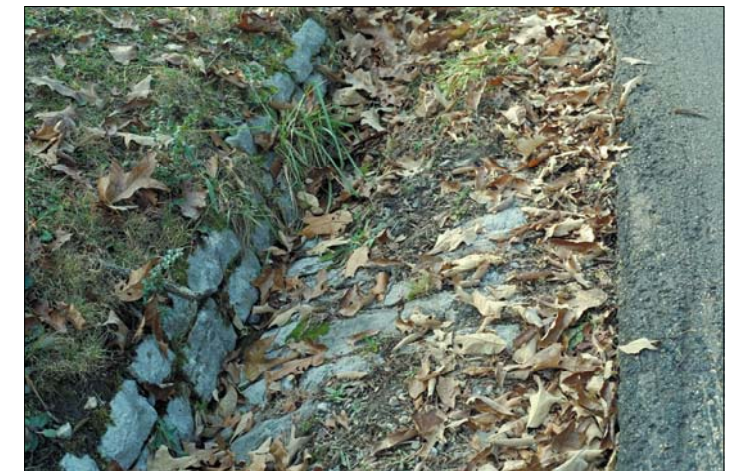
Location of all remaining remnant stone-lined drainage ditches should be documented.
