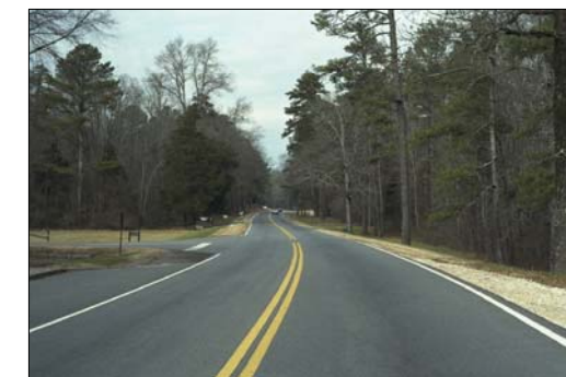
Existing character of LaFayette Road near Brotherton Field.
