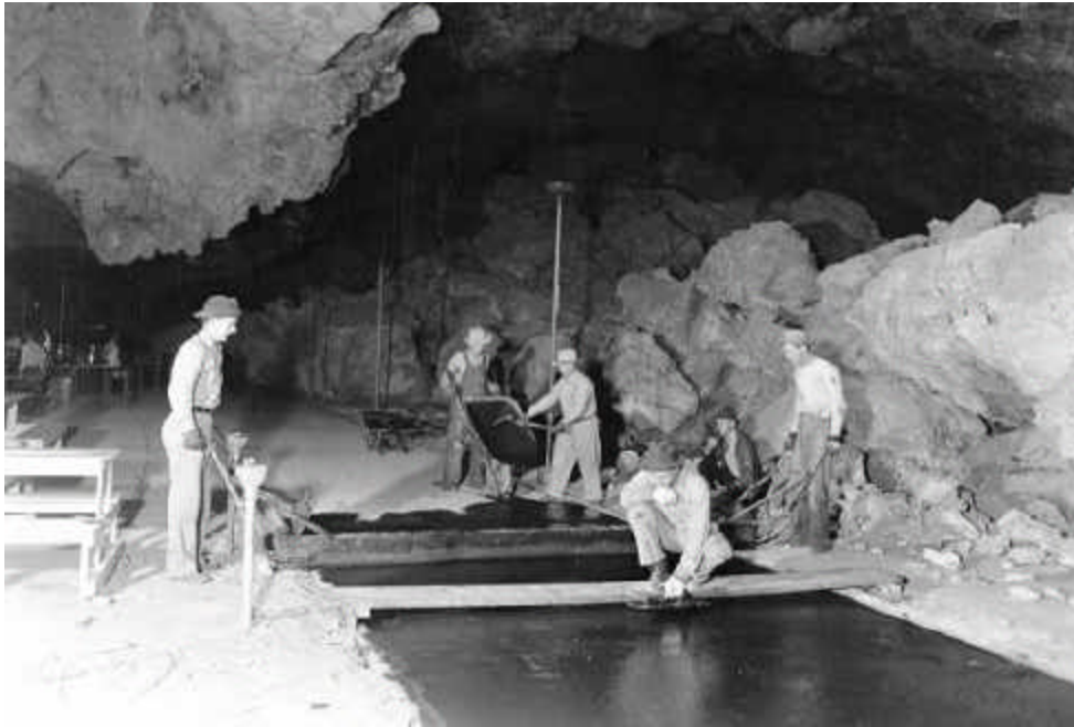
Figure 8. Rattlesnake Springs Camp (Carlsbad Caverns National Park) CCC workers resurfacing floor in the Underground Lunchroom in the late 1930s.
