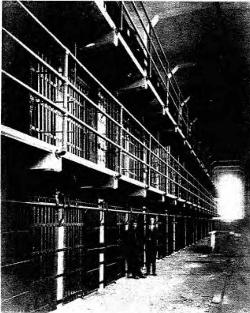
16. Interior of the New Cell House, ca. 1911
