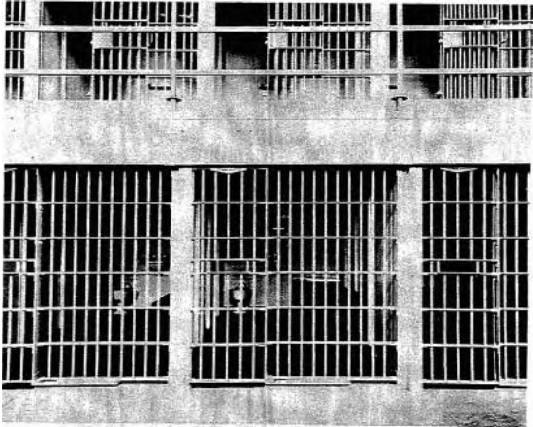
17" Tool-proof Steel Cell Fronts After Remodeling by the Bureau of Prisons, 1934
