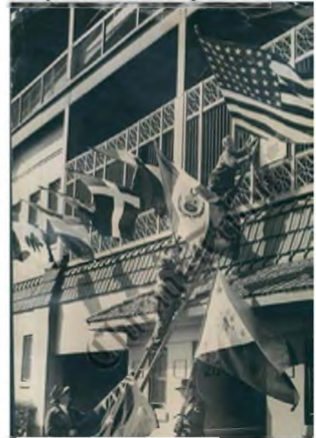
Two mid-1940s photos showing the relationship of the clay tiles to the grilles and steel columns.
