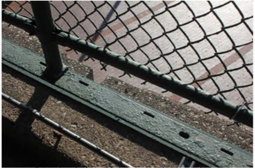
Original angle showing holes for vertical pickets and posts.
